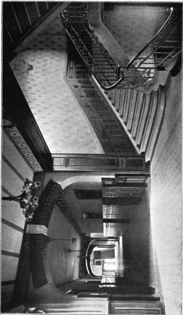
THE SCHOOL OF COMMERCE AT NEUCHÂTEL.—LANDING AND CORRIDOR.
