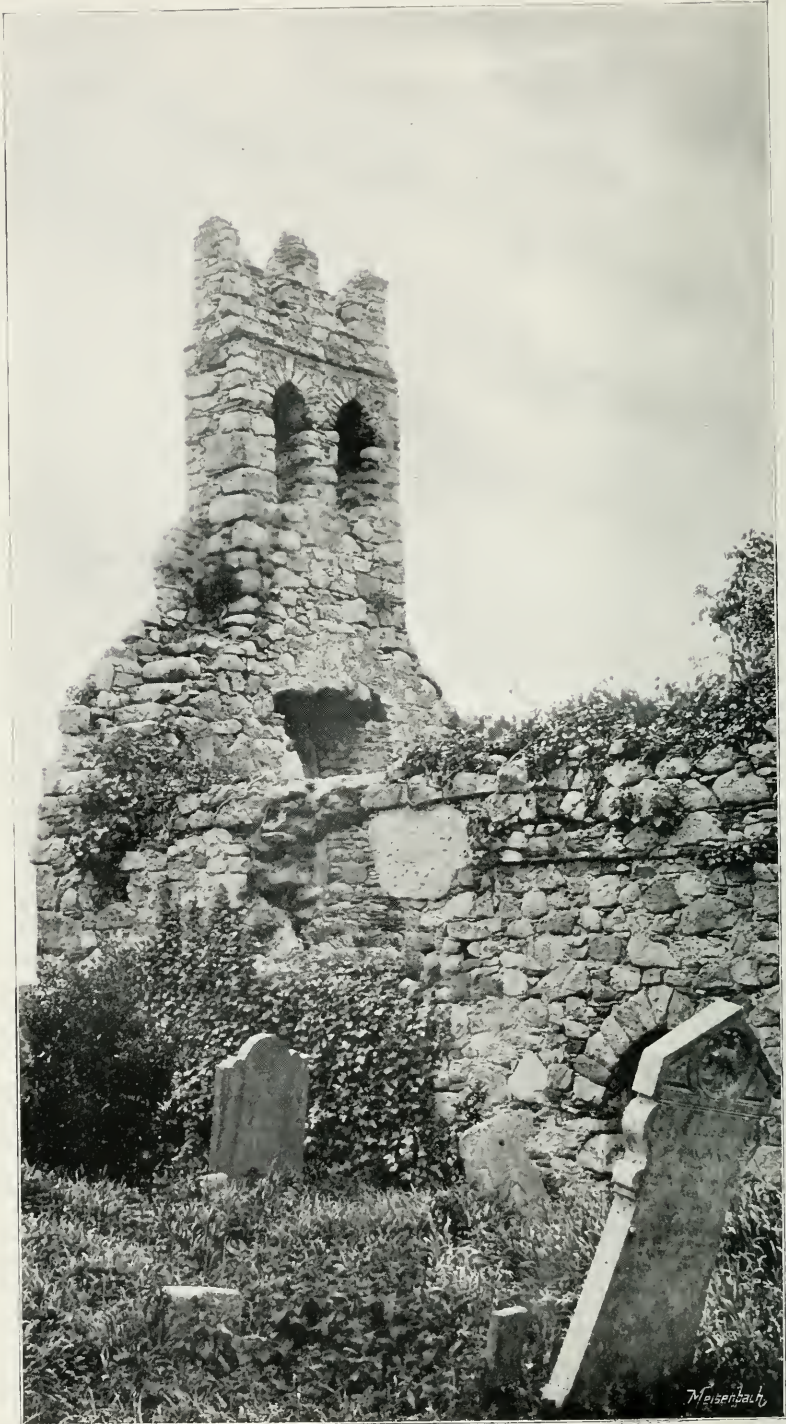
Ruined Church of Dalkey. From a Photograph by Edward Bradford.
