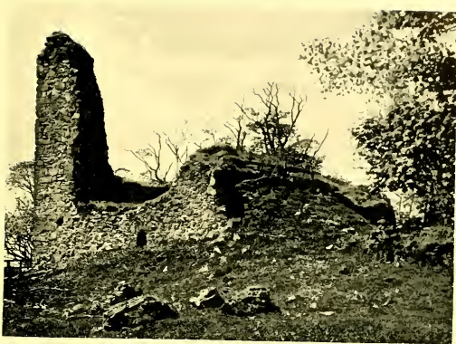
LOCHWOOD TOWER, DUMFRIES.
